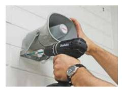
Exclusive design incorporates a dog leg mounting bracket which eliminates the need to separate the horn from the bracket during installation. A real time & money saver!
